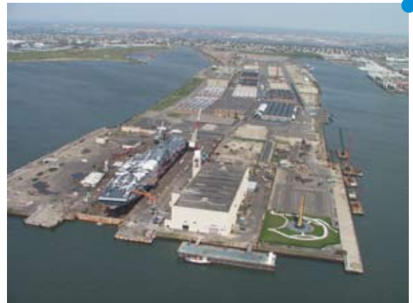
MOTBY redevelopment site
