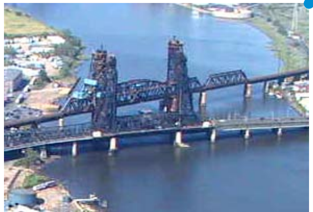
Wittpenn Bridge, crossing the Hackensack River
