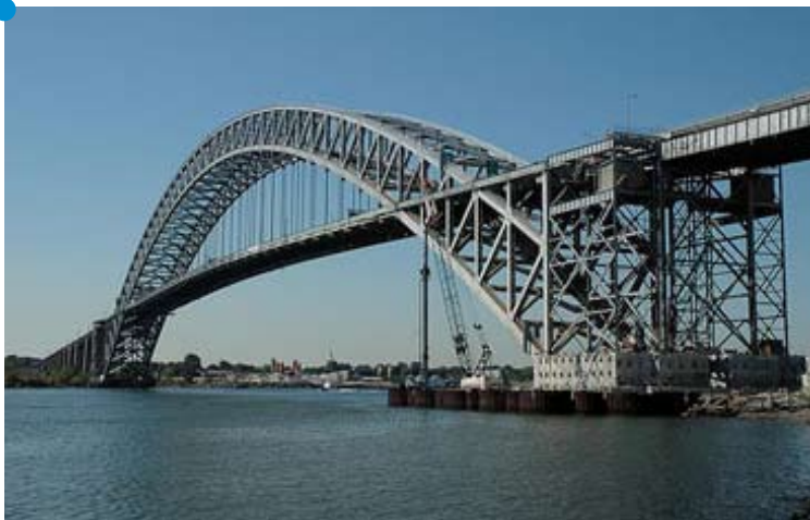
Bayonne Bridge over the Kill Van Kull
