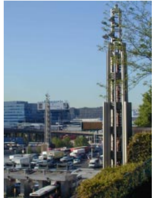
Figure 3.5.2 - Current entrance to the Lincoln Tunnel
