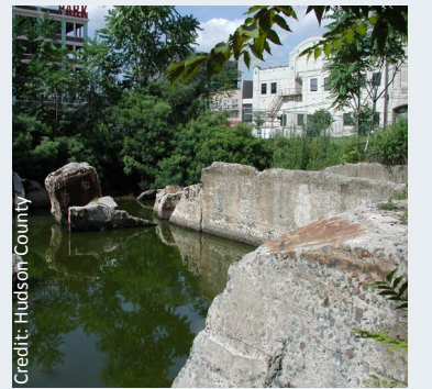
Hoboken/Weehawken Cove prior to walkway construction
