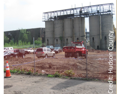
Ground breaking for Berry Lane Park development
