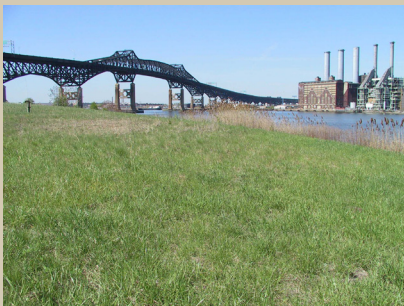
The site of Jersey City's Skyway Park, currently in the planning stages.
