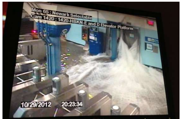
Figure 6 - The floodwaters from the Hudson River entered the PATH subway system through the unprotected elevator shaft.
