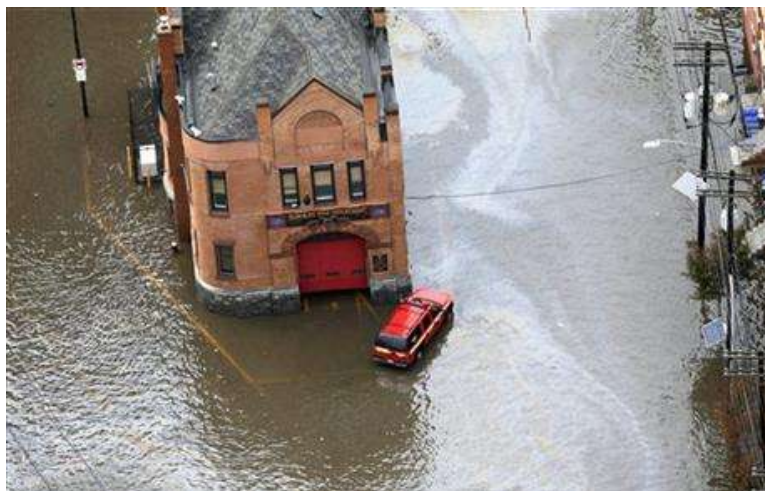
Figure 7 - Hoboken's Fire Headquarters and Fire Stations were flooded during Hurricane Sandy and were abandoned until the waters receded.
