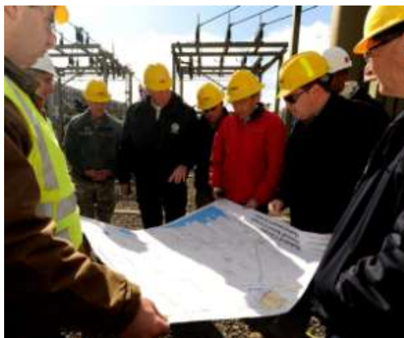
Figure 4 - FEMA Deputy Administrator Rich Serino, second from left, discusses power restoration with U.S. Department of Energy Secretary Chu, red jacket, along with PSEG power engineers.
