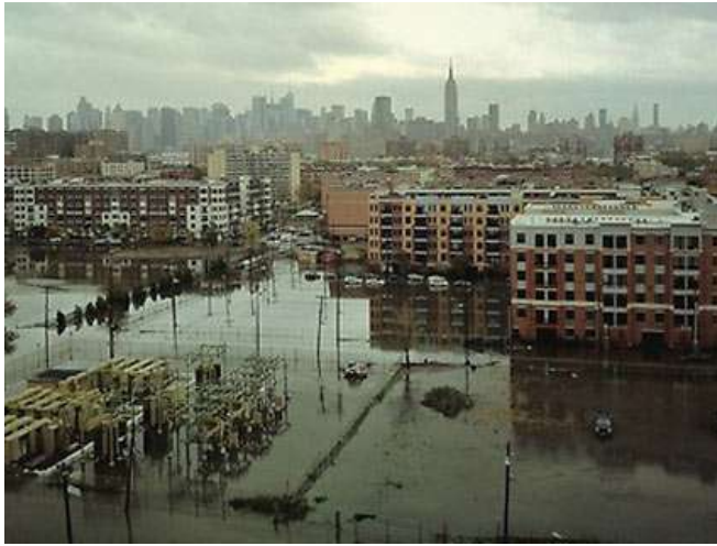
Figure 2 - All three (3) of Hoboken's electrical substations were flooded and damaged during Hurricane Sandy causing widespread power outages for over 10 days.
