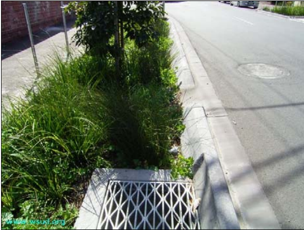
Bioretention swale retro-fit to roadway
