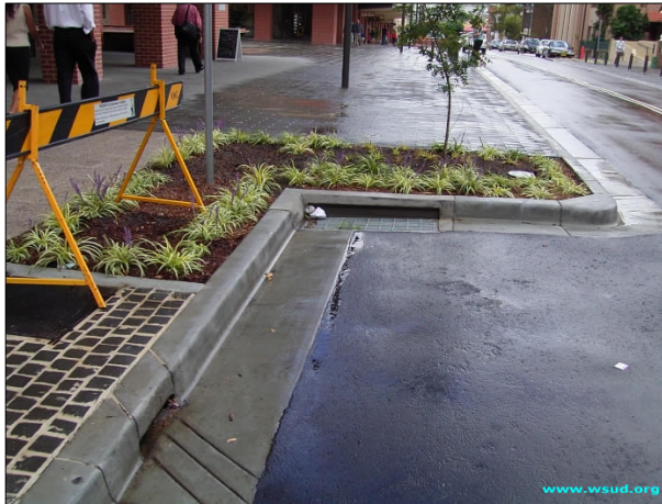
Street Tree stormwater treatment retrofit
