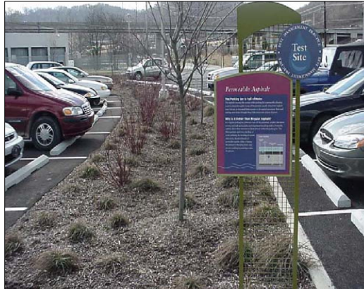
Bioretention swale in a parking area
