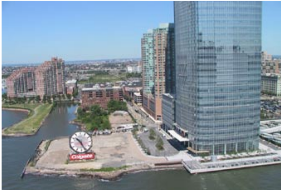
Veteran's Park Gap Site, Jersey City
