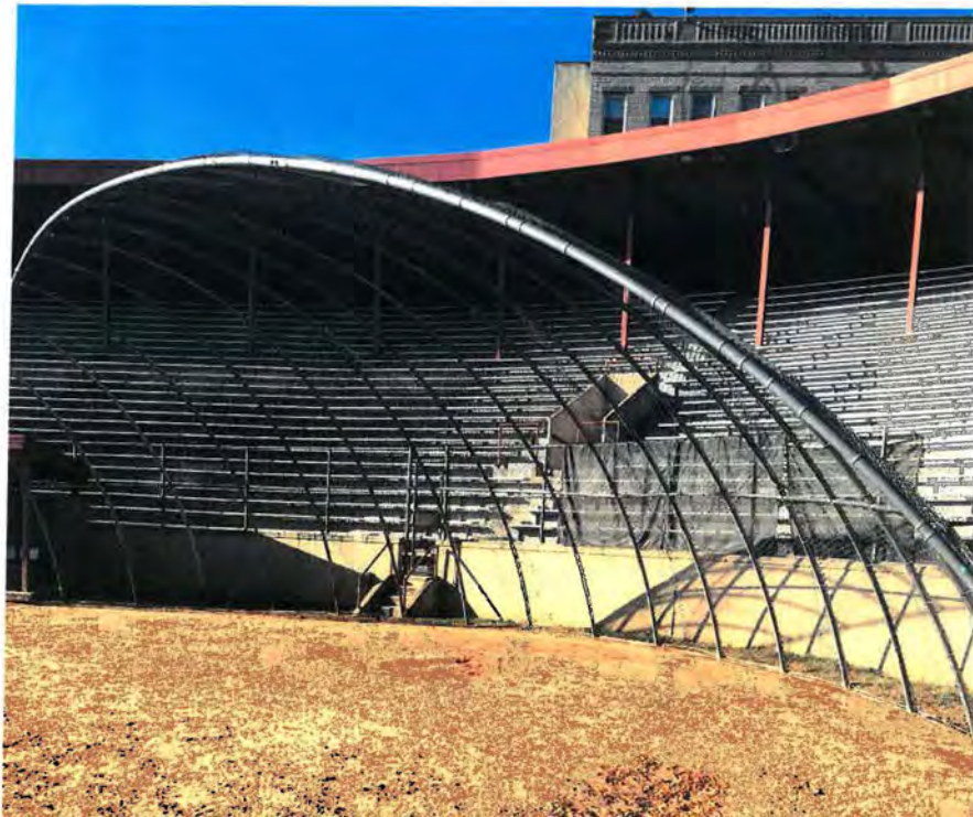
Miller Stadium Field Surface Improvements Existing Conditions - Backstop
