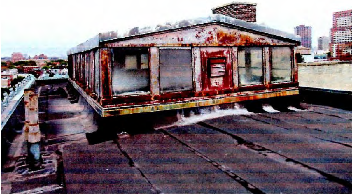
Main Library Roof Restoration Existing Conditions - Ornamental Copper Cresting
