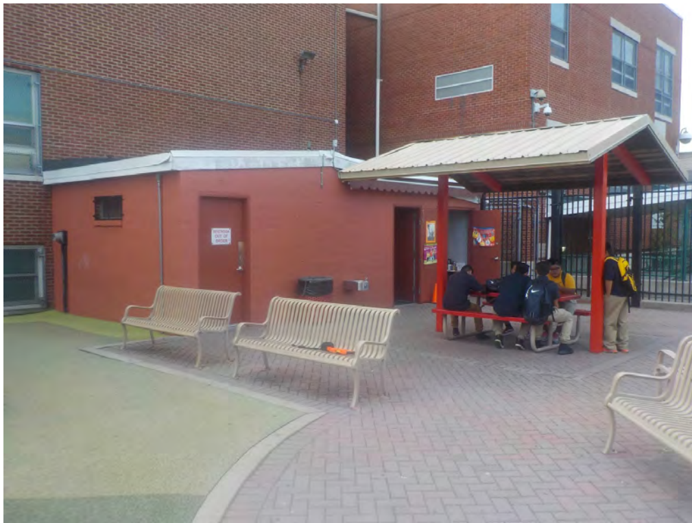
Veteran's Park Improvements Existing Conditions - Picnic Tables
