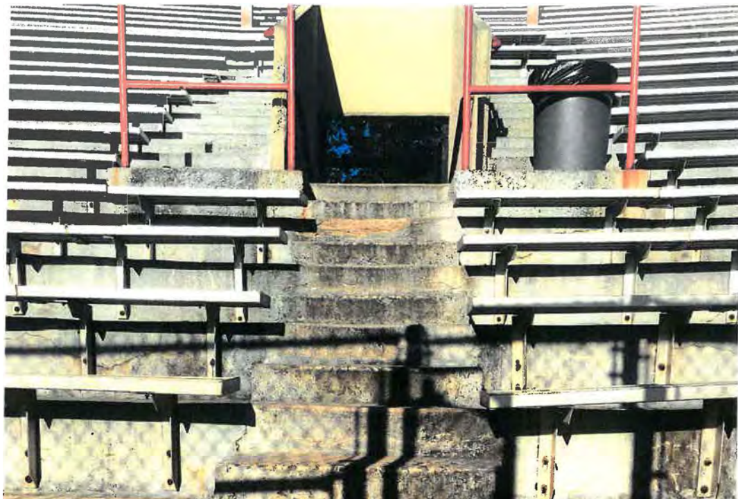
Miller Stadium Field Surface Improvements Existing Conditions - Bleachers
