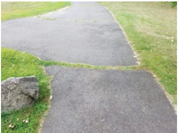
12B - Paved walkway, 5 feet wide, cracked.
