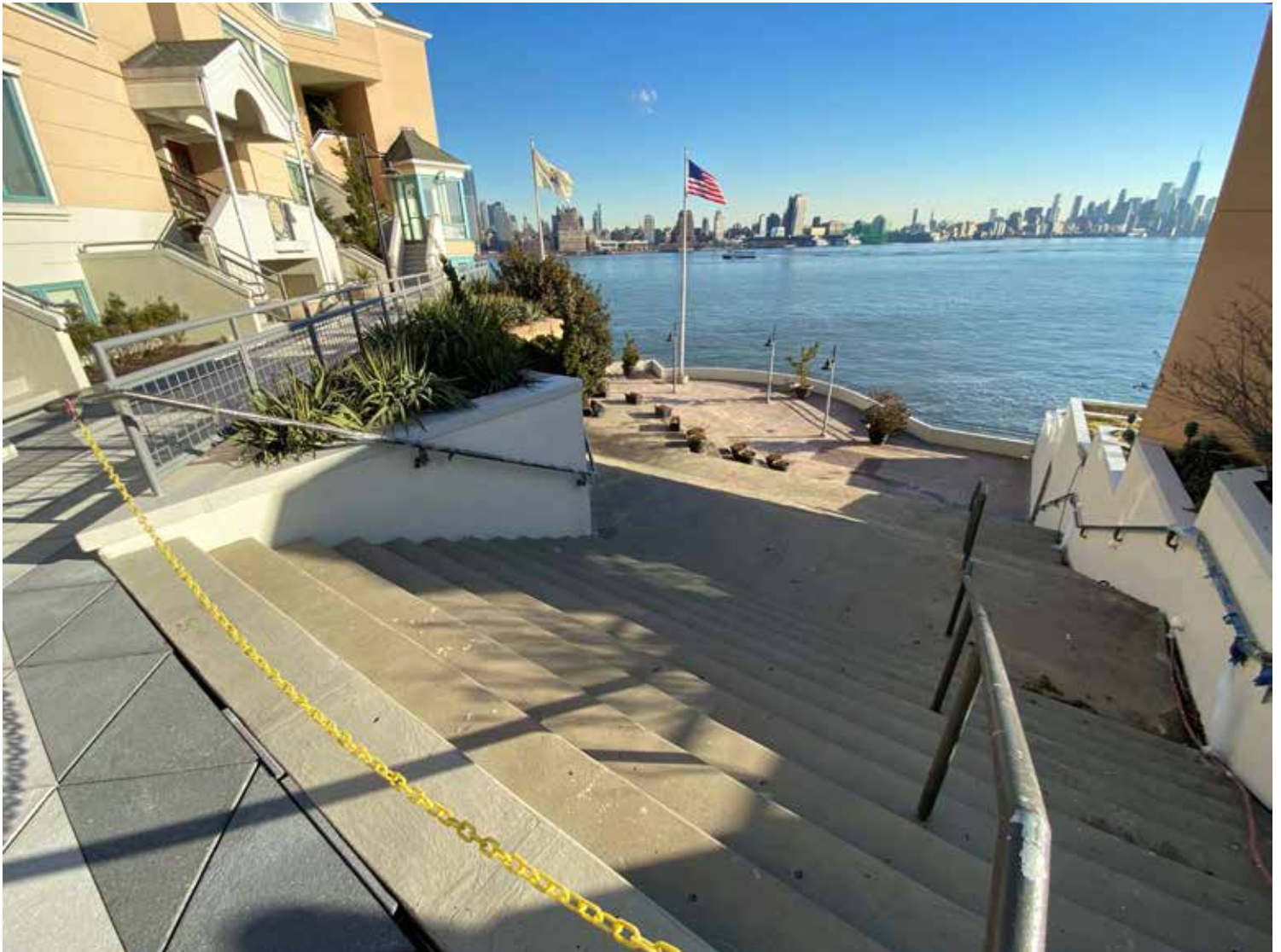
Pictured: Existing conditions
