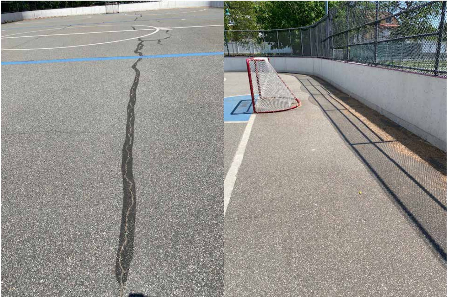
Pictured: Existing conditions
