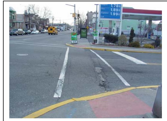
View northbound across 76 th Street east side of JFK
