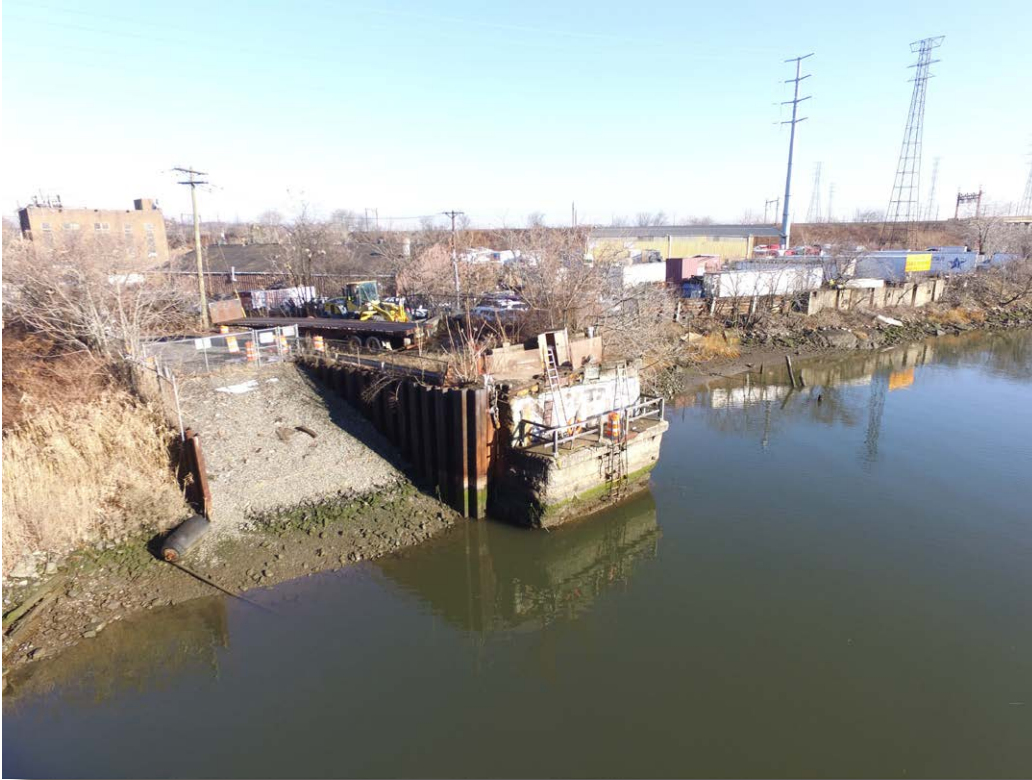
Plate 1: West abutment for the 1911 Newark Turnpike Bridge, predecessor of the 1930 Wittpenn Bridge.
