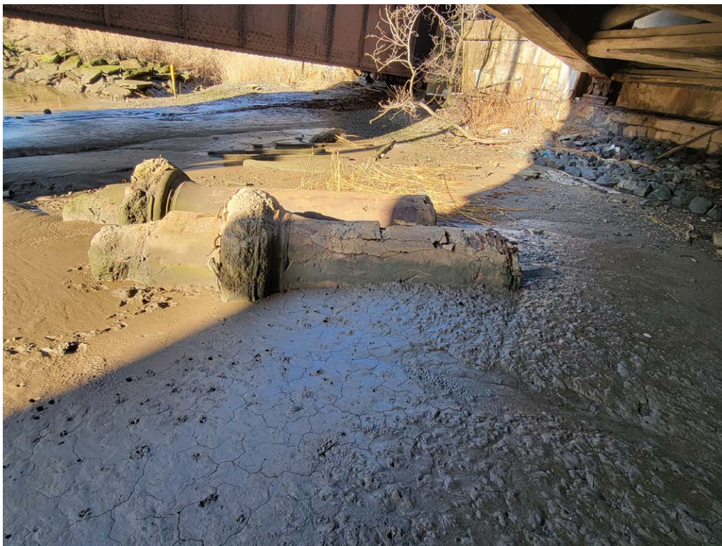
Plate 5: Unidentified architectural concrete columns or piers located beneath the 1930 Wittpenn Bridge.
