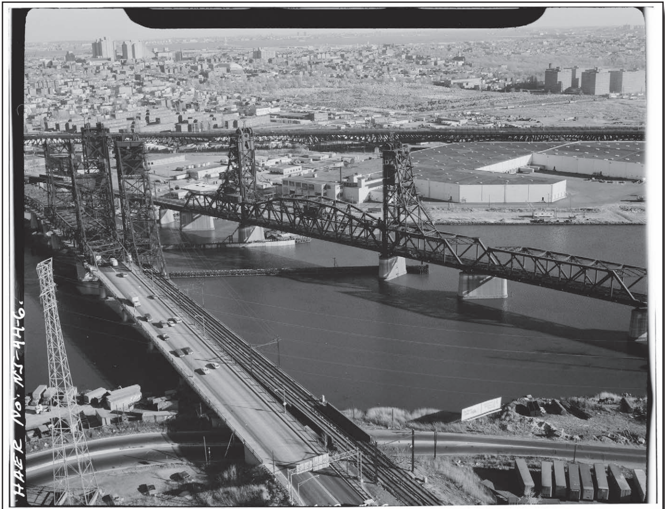
Figure 19: Bridges connecting Kearny and Jersey City, view southeast. The 1930 Wittpenn Bridge is on the left, with Pennsylvania Railroad Harsimus Branch Bridge immediately on its right. To the far right is the Pennsylvania Railroad PATH Bridge. In the background is the Pulaski Skyway (Boucher 1978; Photograph NJ-44-6 from HAER NJ-44, PATH Transit System Bridge Looking Southeast; Courtesy of the Library of Congress).
