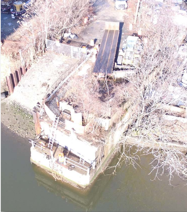
Plate 3: West abutment for the 1911 Newark Turnpike Bridge, predecessor of the 1930 Wittpenn Bridge.
