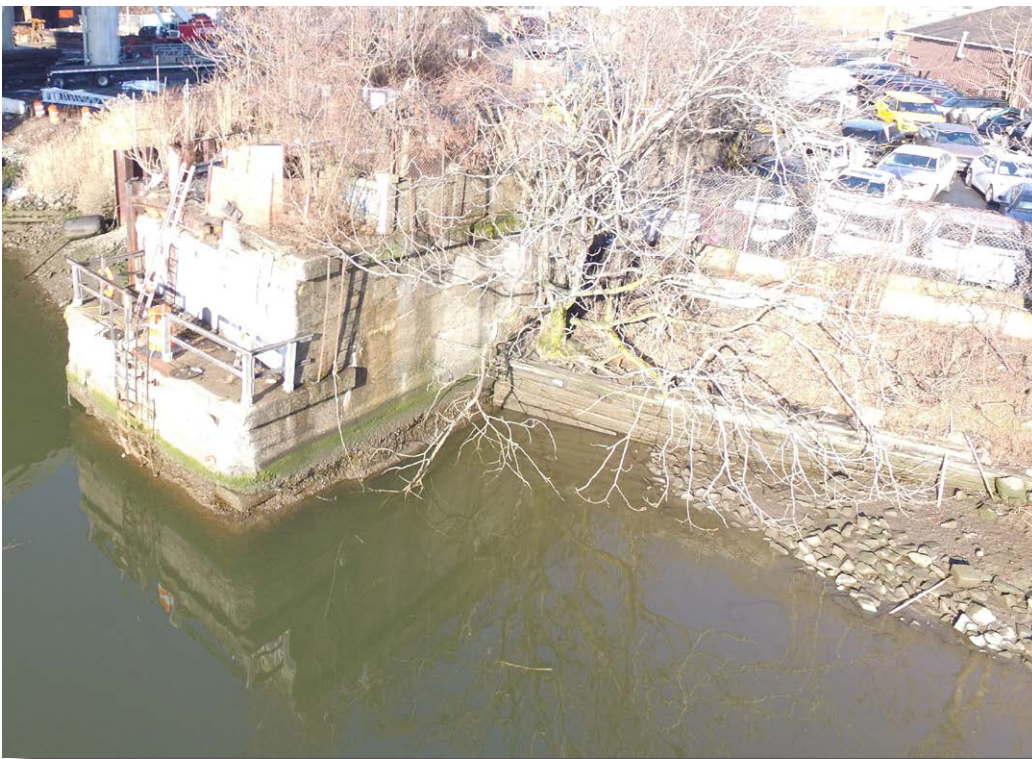
Plate 2: West abutment for the 1911 Newark Turnpike Bridge, predecessor of the 1930 Wittpenn Bridge.
