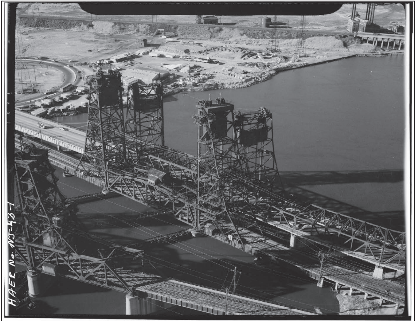
Figure 20: Bridges connecting Kearny and Jersey City, view northwest.
