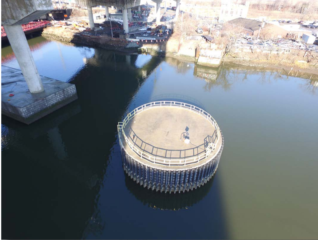
Plate 4: Concrete and steel plate pylon, which is part of the Pier Protection System for the 2021 Wittpenn Bridge, in the approximate location as the pivot pier (once associated with the 1911 Newark Turnpike Bridge).
