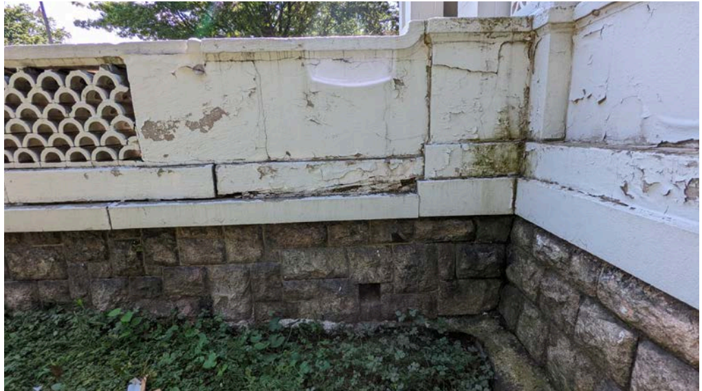
19. Fieldston base and damaged concrete and terra cotta wall
