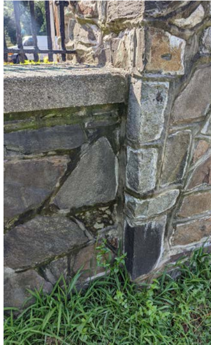
35. Detail showing different pointing campaigns with biological growth and damaged pointing
