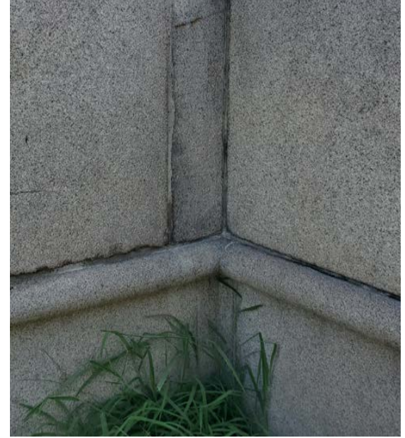
9. Detail of wall at rear of statue; typical condition of mortar joints
