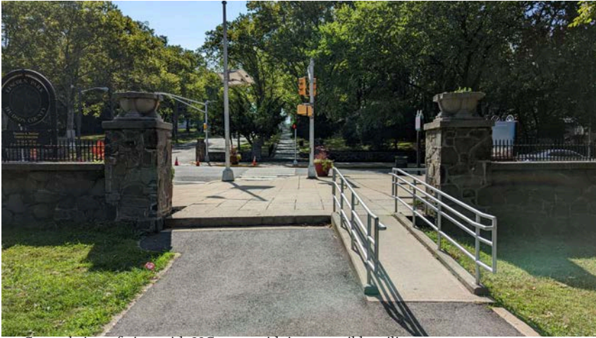
37. General view of piers with HC ramp with incompatible railing
