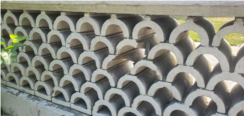
29. Detail of damage to the existing walls (decorative arches are painted terra cotta)
