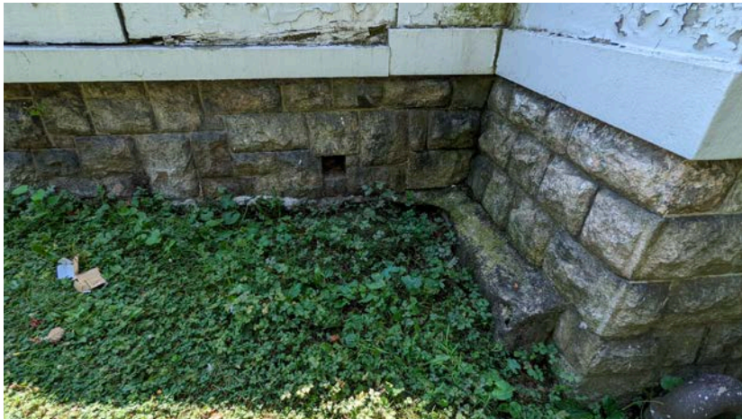
15. Fieldstone base showing soiling and missing pointing
