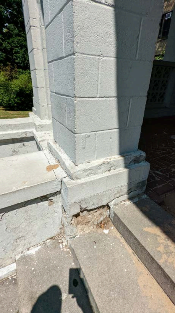
17. Spalling at original stone base of replaced column
