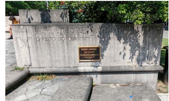
3. Low granite wall with text and art deco carvings; note staining
