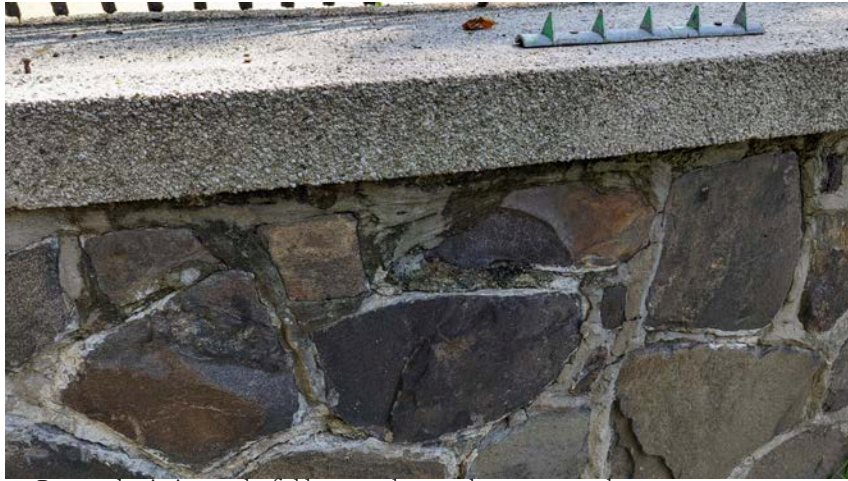
43. Damaged pointing on the fieldstone and exposed aggregate on the cast stone cap
