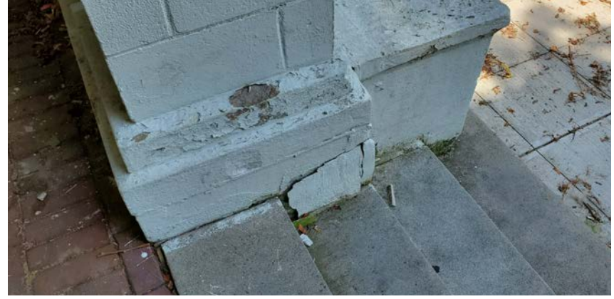
25. Freeze thaw damage at original stone base
