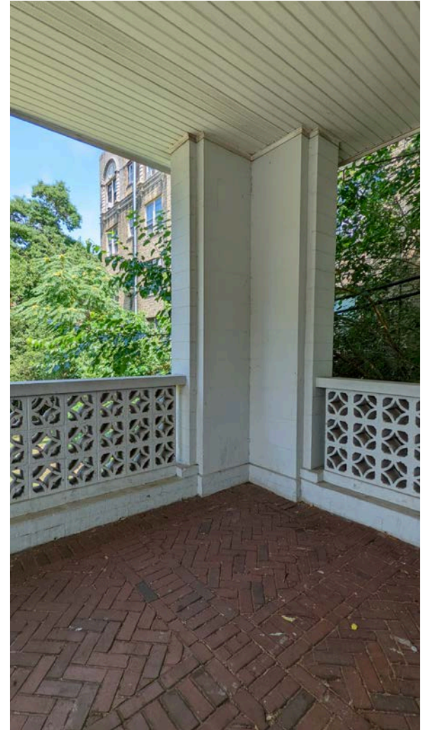
16. CMU corner pier and railings that were constructed in the 1970's renovation
