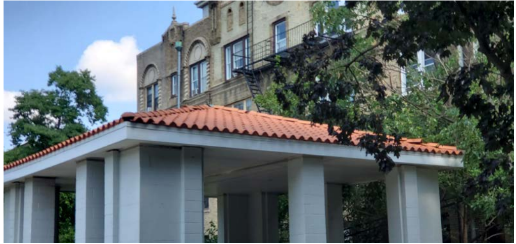
18. Terra cotta roof; several tiles are missing
