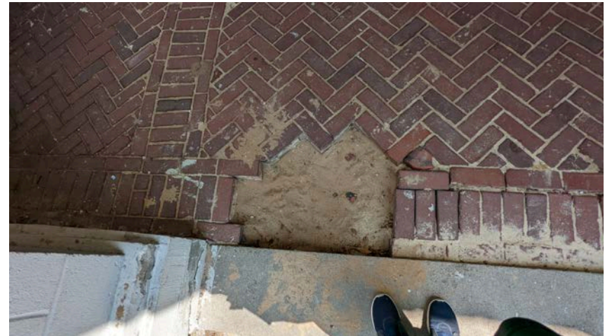
13. Missing brick at interior floor
