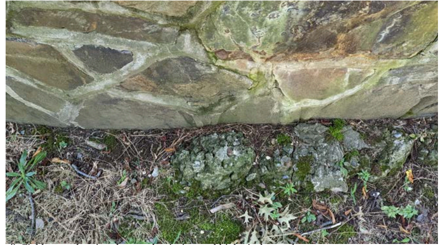
38. Fieldstone showing damaged pointing and biological growth staining
