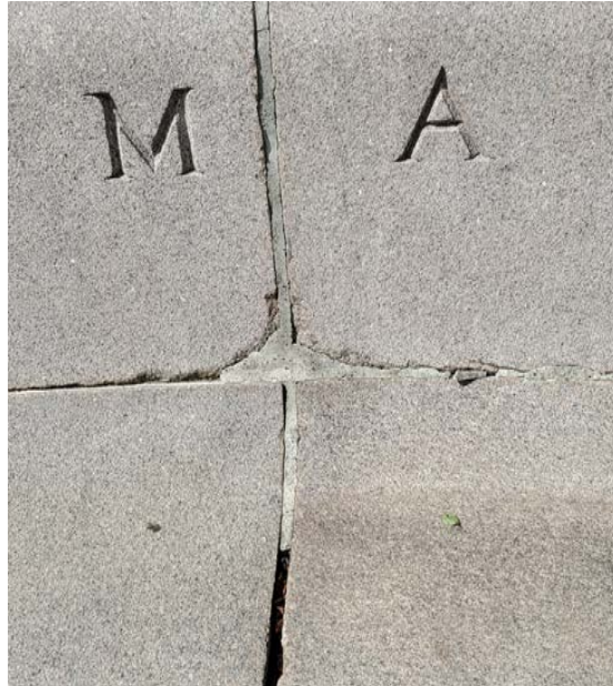
8. Closeup of paving showing need for careful repointing
