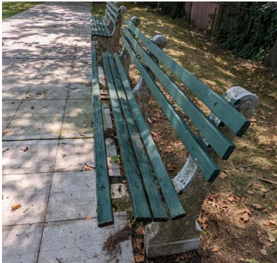
1. Damaged concrete and wood slat bench
