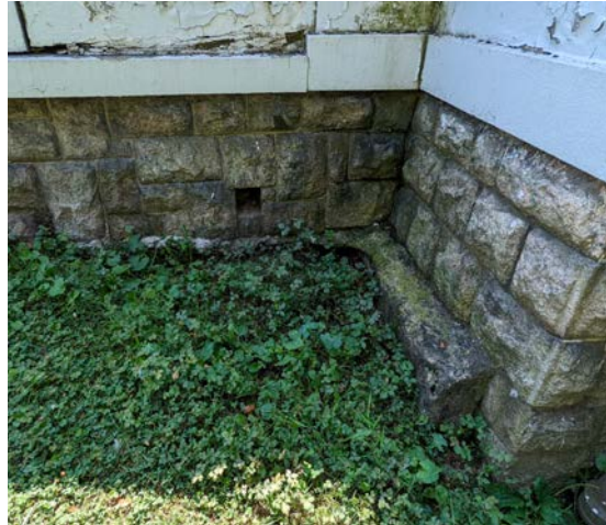
21. Stone base of the Summer House; clear plant growth, clean masonry and repoint as needed
