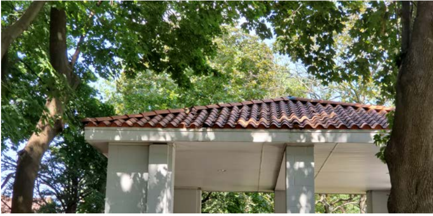
24. Terra cotta roof is missing several tiles but is in overall good condition
