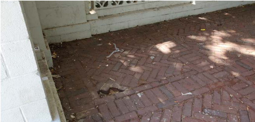
26. Brick floor with several missing pavers
